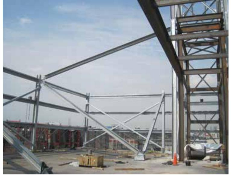
Superbrace framing system for the steel beacon tower.
