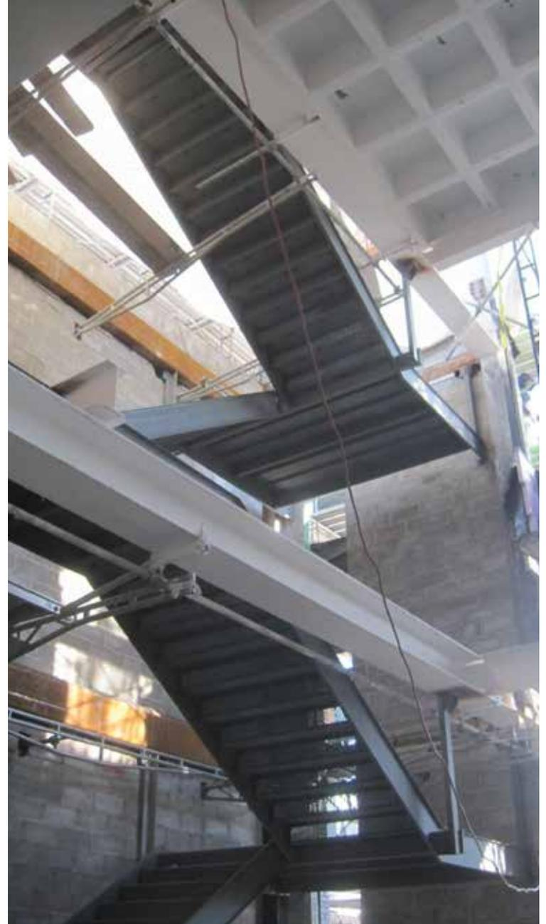
View of the new architectural stair from the ground floor. Underside of the concrete waffle slab is visible on the right.
