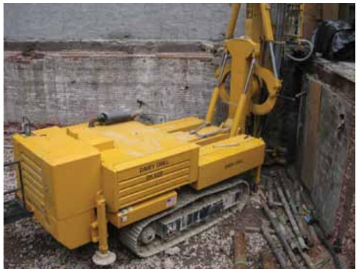
Figure 3: The micro-pile rig. The width of the rig limited how close its drill mechanism could get to the face of the building.
