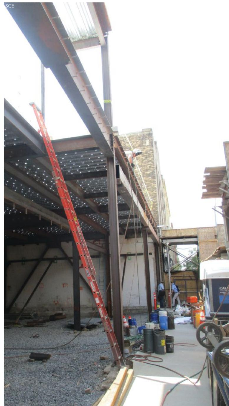
“floor” was constructed of galvanized metal grating secured with mechanical fasteners.
