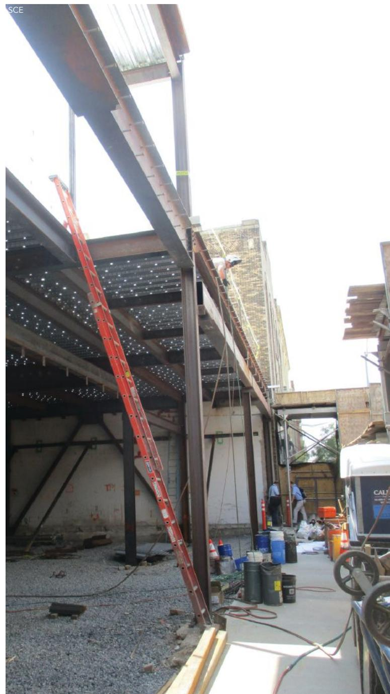
“floor” was constructed of galvanized metal grating secured with mechanical fasteners.
