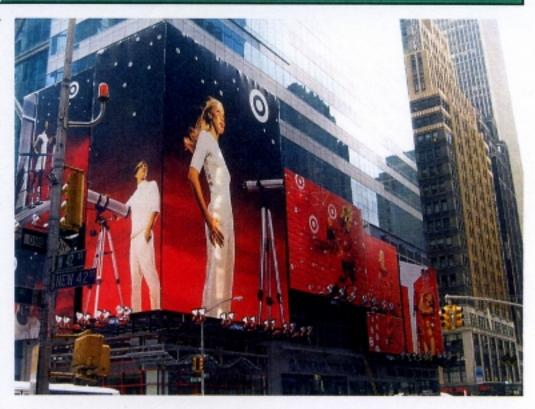
The signs at the two northern corners required double cantilevers that could work independently from each other. The southern face, which had no primary steel tube, required the team to support the signage structure directly through building stub-outs.
